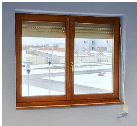
Standard double-glazing window 4/16/4 in CIRCE building
